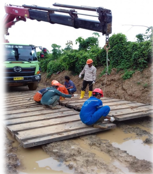
gripper access without civil works preparation
